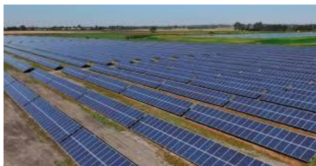
Solar Farm in Day Lane
